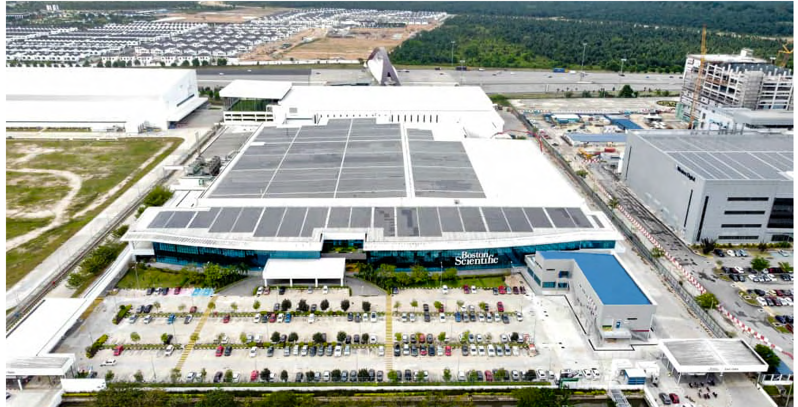
In 2023, we completed installation of solar panels in our Penang manufacturing site. This is currently our largest solar installation.
